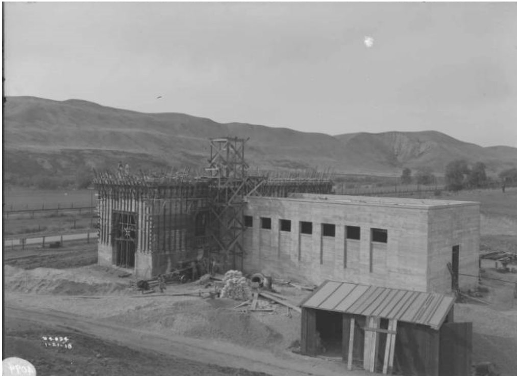
Figure 6: Capistrano Substation under construction, January 21, 1918.
