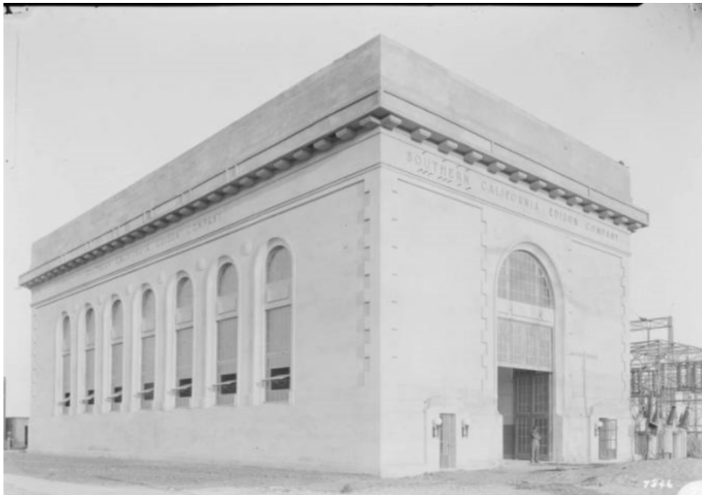
Figure 24: SCE Vestal Substation, Richgrove, California, 1921.
