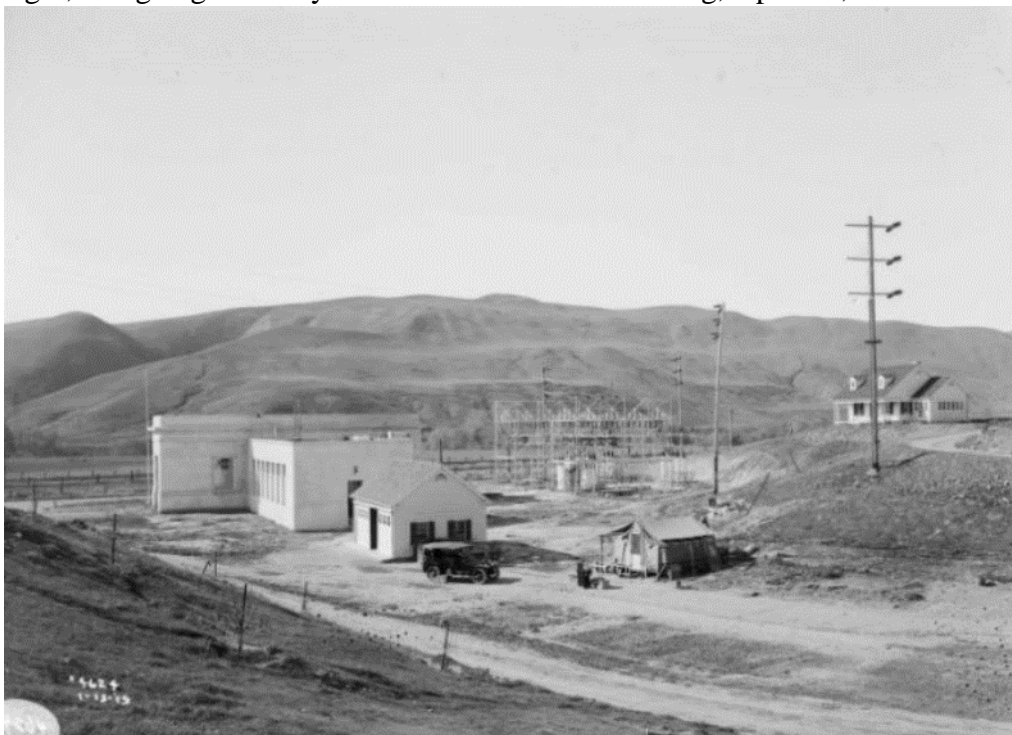
Figure 11: Capistrano Substation from the same angle after completion, January 13, 1919.
