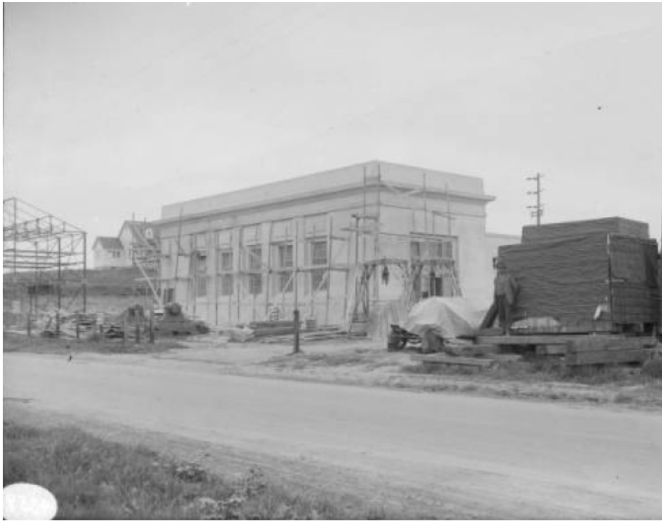
Figure 12: Capistrano Substation under construction from Camino Capistrano, 1918.
