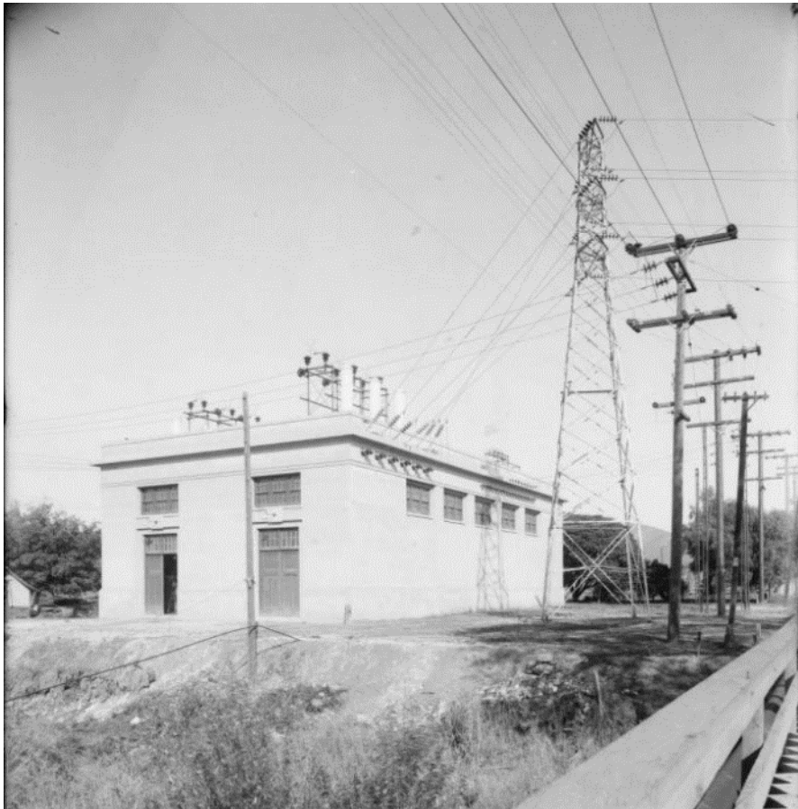
Figure 25: SCE Puente Substation, 1913.
