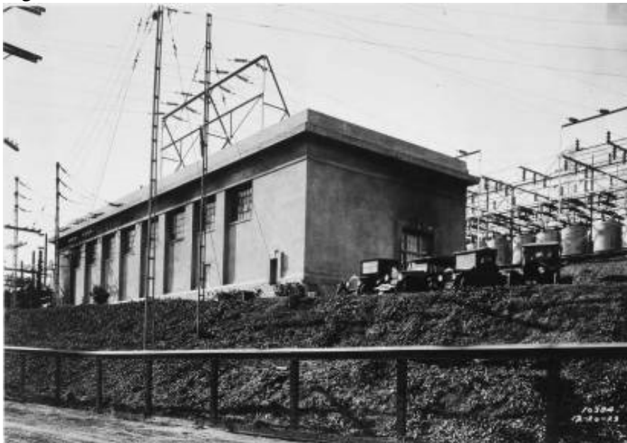
Figure 26: SCE Colton Substation, December 20, 1923.
