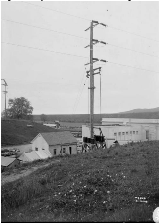
Figure 9: Wood transmission pole with incoming line, garage, and substation, April 10, 1918.
