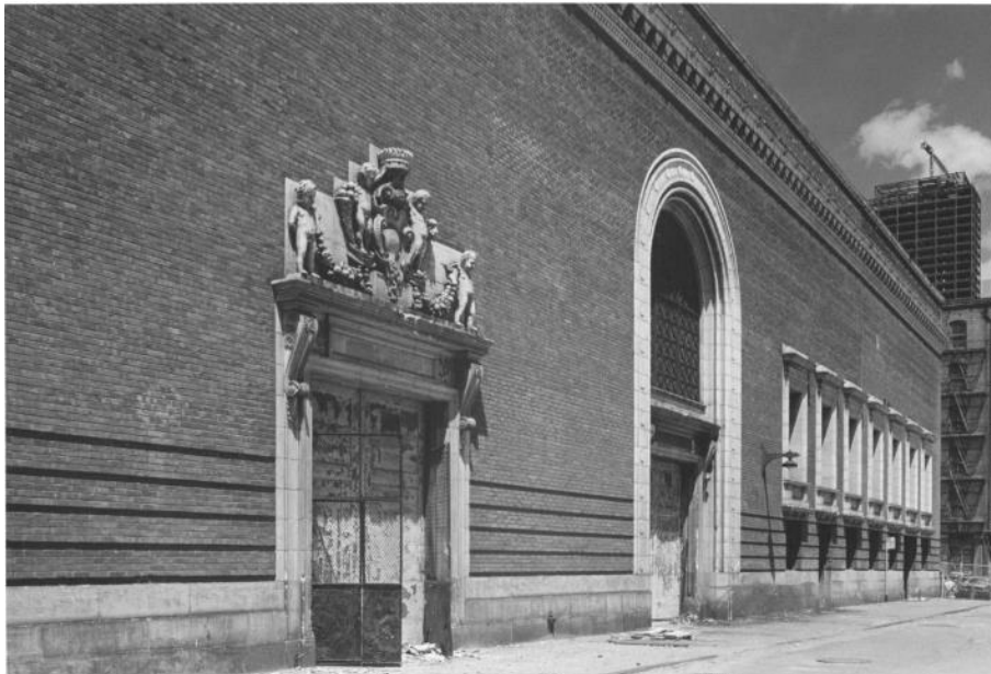
Figure 22: PG&E Jessie Street Substation, San Francisco, April 22, 1974.
